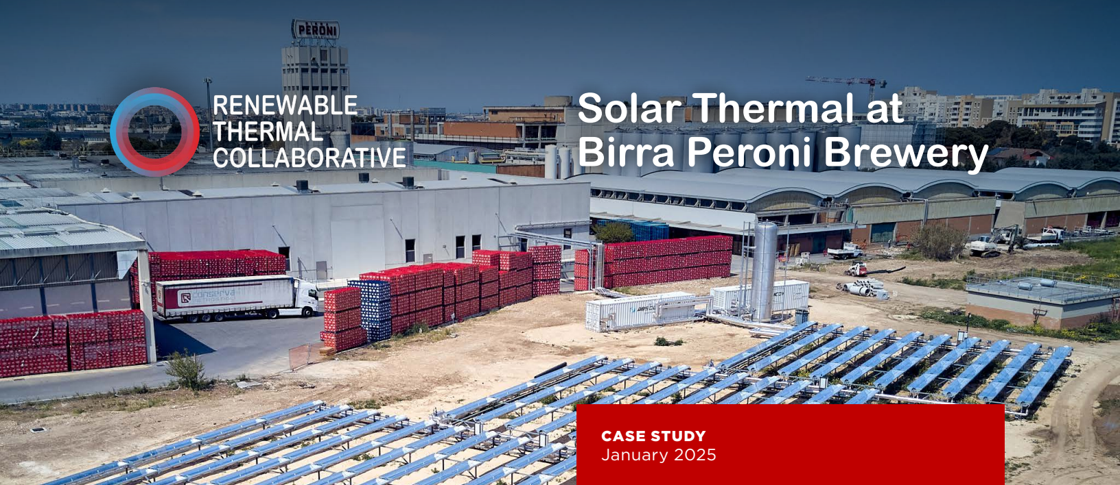
Solar thermal field at the Birra Peroni brewery in Bari, Italy Credit: Antonio Tartaglione
